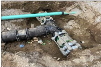
Installing the 36-inch by 20-inch Tee on Section 23 for Emergency Interconnection
