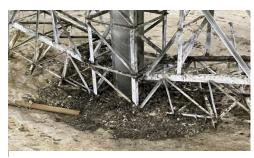
Figure 3. Gravity Thickening Center Column Clog
